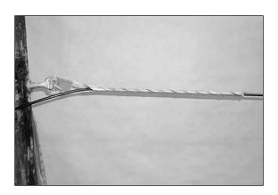
FIBERLIGN® Lite Tension Dead-end for All Dielectric Self-Supporting (ADSS) Fiber Optic Cable Installed
